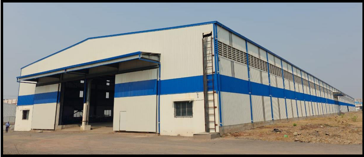
(Pre-Engineered Building built by us for a client at Umbergoan, Gujarat)
