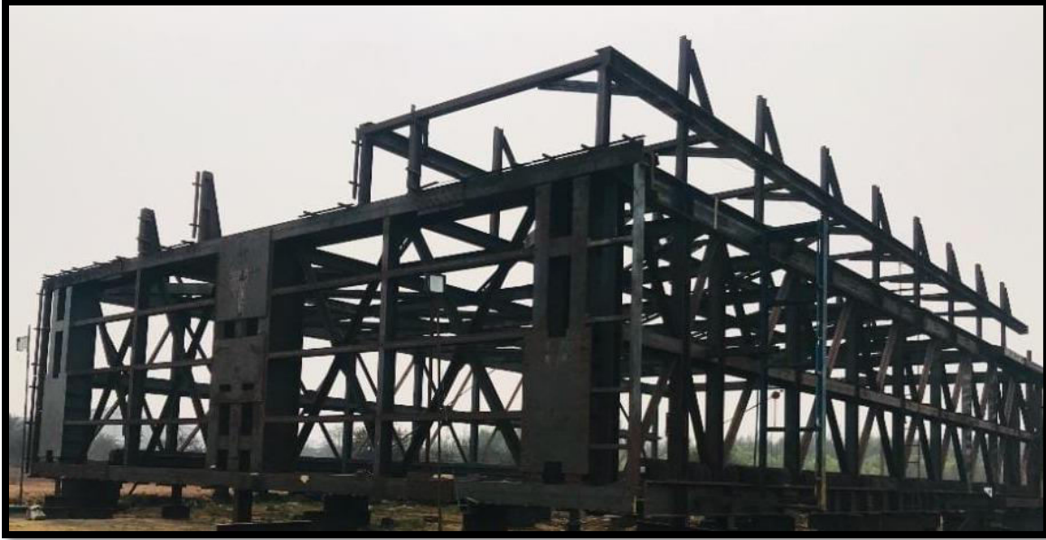
(Accumalator Structure built by us for John Cockerill India Limited)
