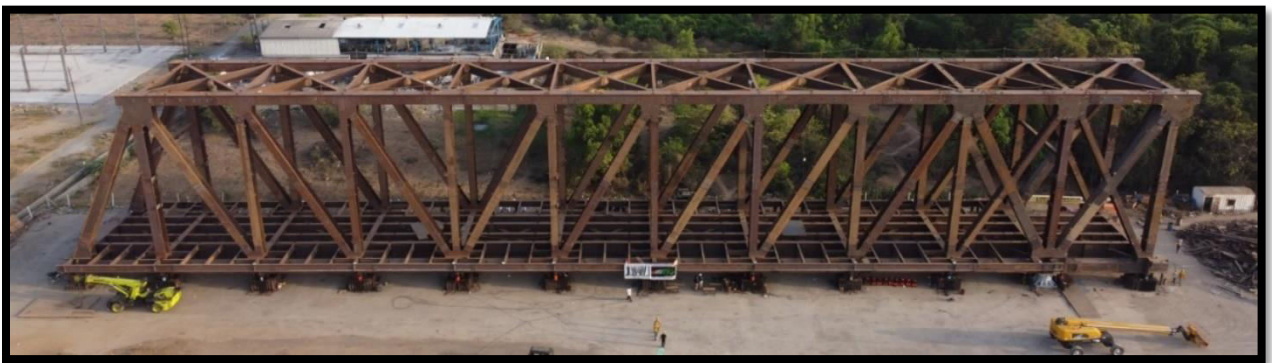
(Steel bridge structure built by us for the Mumbai-Ahmedabad High-Speed Rail (MAHSR) project)
